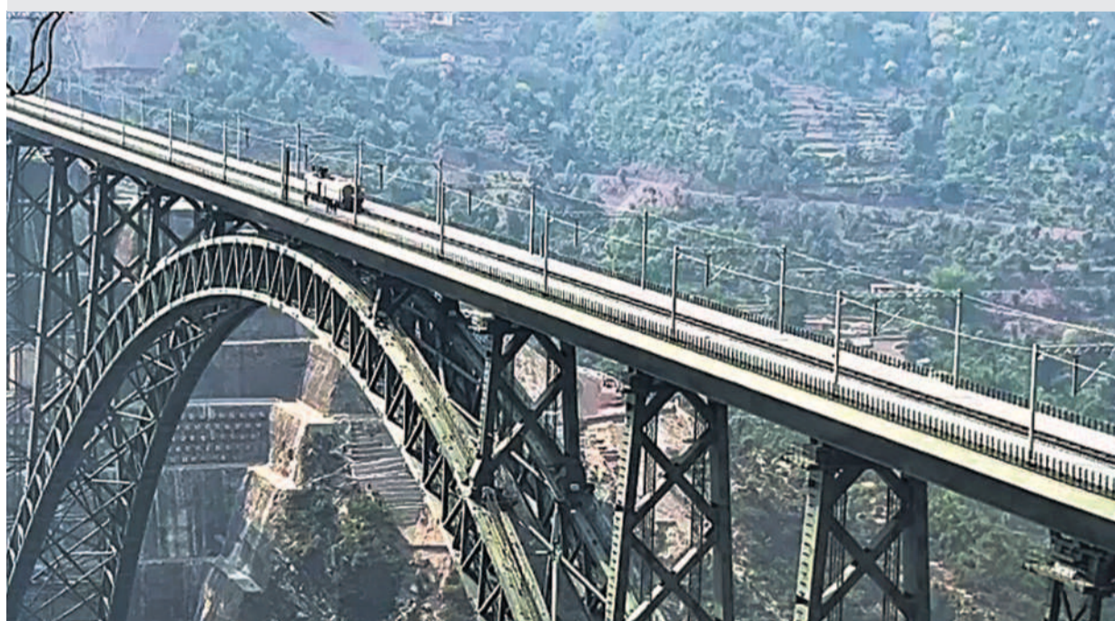
The railways on Sunday successfully conducted an electric engine trial on the newly constructed world's highest railway bridge — Chenab Rail Bridge — built between Sangaldan in Ramban district and Reasi, Jammu and Kashmir. — Photo: ANI
